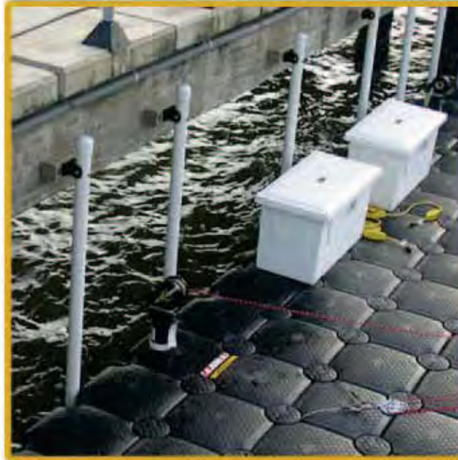
CALM WATER MOORING USING TIDE MANAGER SYSTEM
