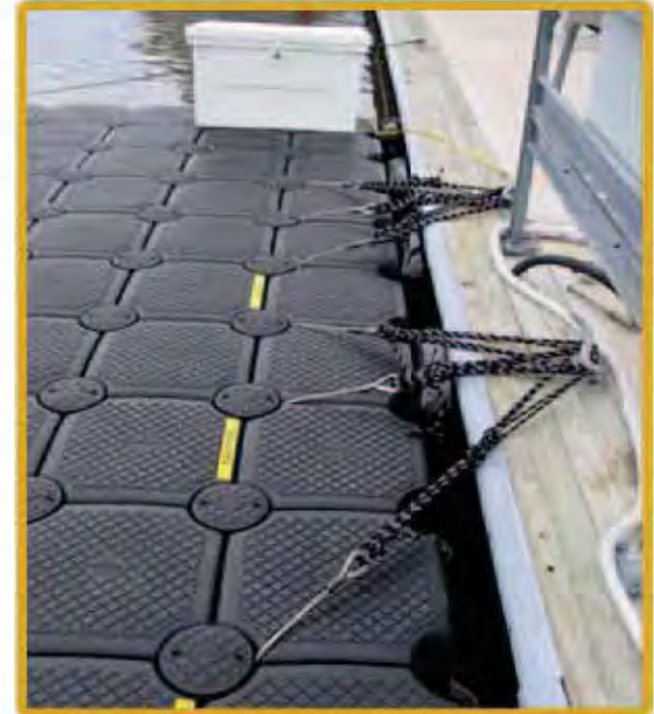
FLOATING DOCK MOORING USING IN-DECK CABLE SYSTEM
