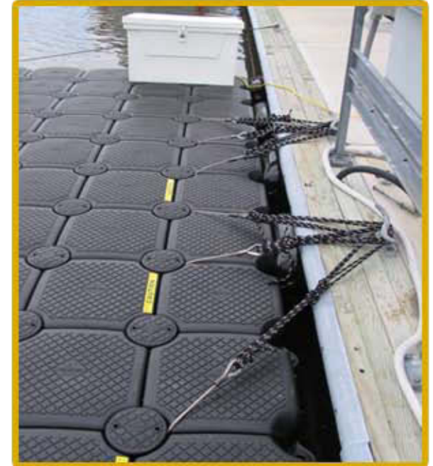
FLOATING DOCK MOORING USING IN-DECK CABLE SYSTEM
