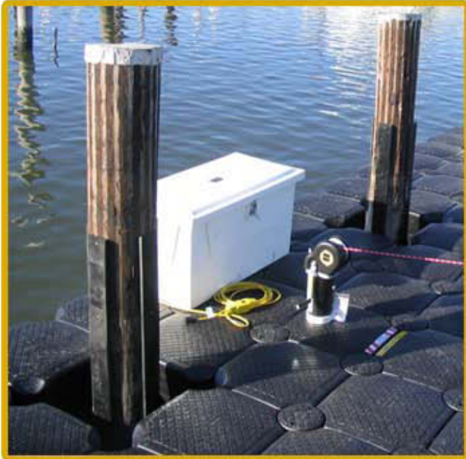
ROUGH WATER MOORING USING INTEGRATED PILINGS
