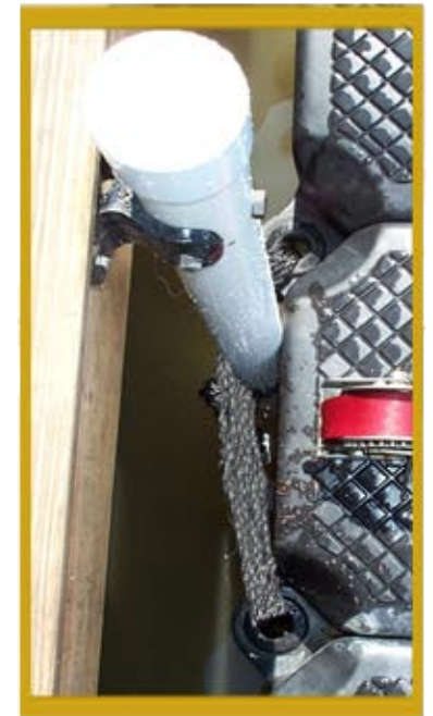
Mooring pole tied to the Jet Dock
