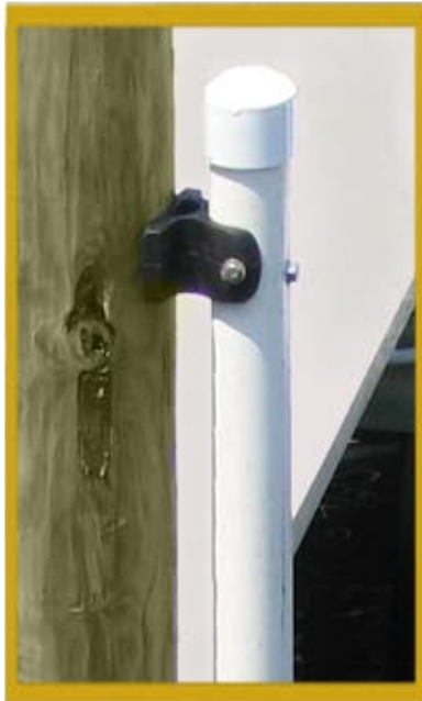
Mooring Bracket attached to a piling
