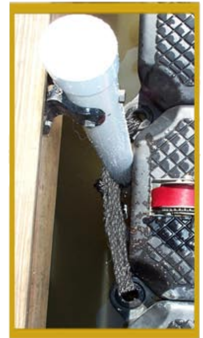
Mooring pole tied to the Jet Dock
